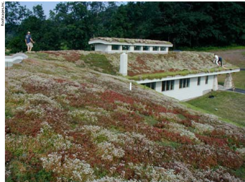
The Life Expressions Center, a chiropractic center in Pennsylvania designed a decade ago, was planted with 6,000 sedum plants that help reduce summer heat radiation and storm water runoff.
